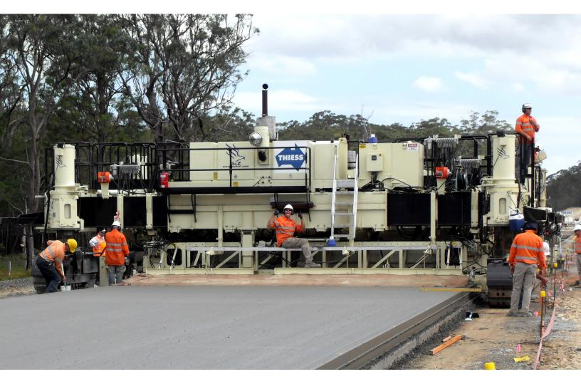
The S1500 Slipform Paver is the largest paver offered by G&Z. Its stout design makes it capable of meeting the strictest smoothness specifications at wide multiple-lane paving applications. The S1500 features a telescopic tractor frame, telescopic front walkway, and a hose tray that can telescope from 18' (5.5m) to 42' (12.8m), the largest in the industry. Its time tested and proven design makes the S1500 the paver of choice for multiple-lane mainline and airport work.
